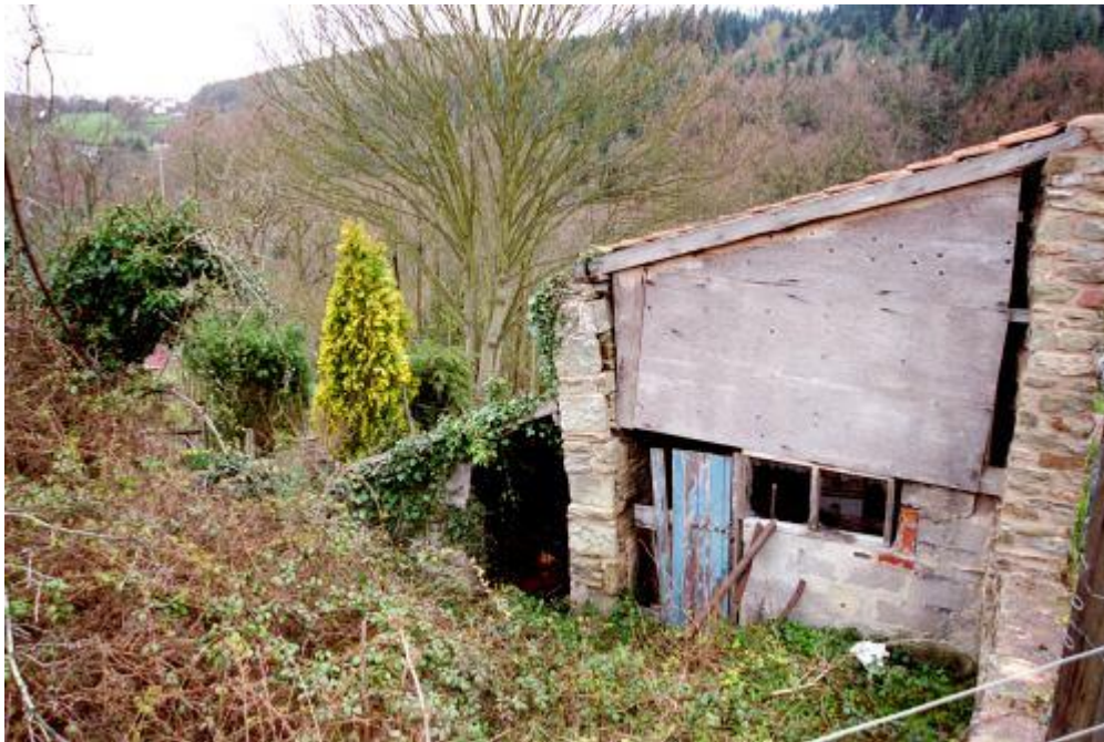
An old building associated with the colliery (SO 605 154) looking north
