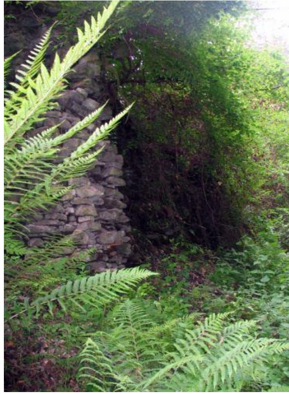
Stone bridge abutments, looking SW
