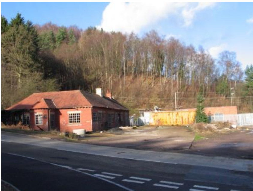
Related buildings with the disused tip in the background, looking NNW
