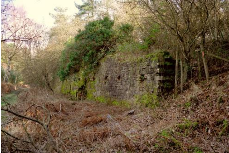
Colliery building remains before clearance
