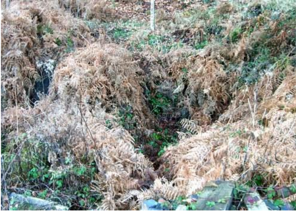
A closer view of the collapsed level entrance
