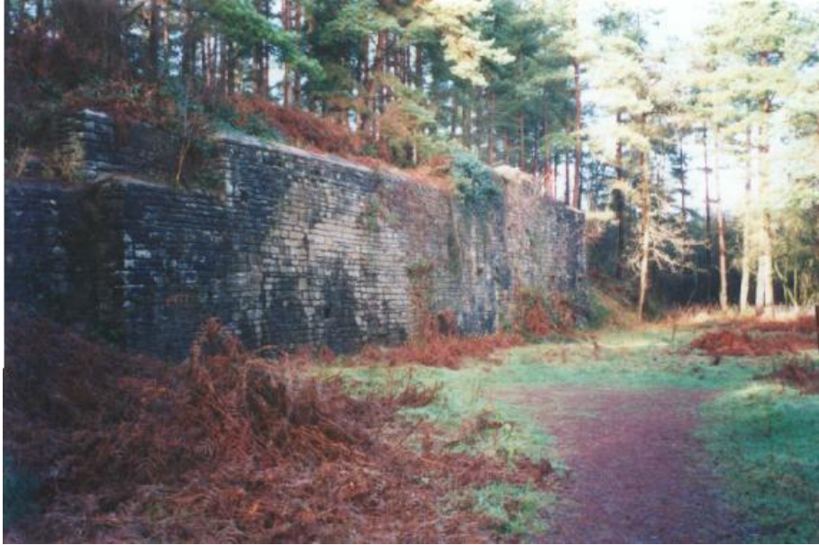
Site of screens, looking N
