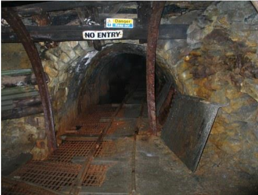
The interior of the Old Furnace Level
