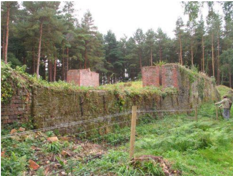
Colliery walls (recent)
