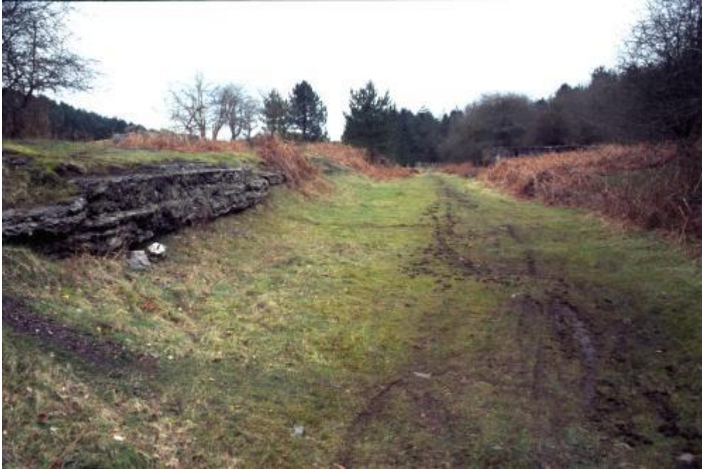
Remains of loading wharf (SO 638 139) looking south
