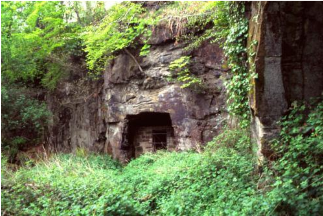
Trafalgar to Strip- and-at-it tunnel entrance (1), looking N
