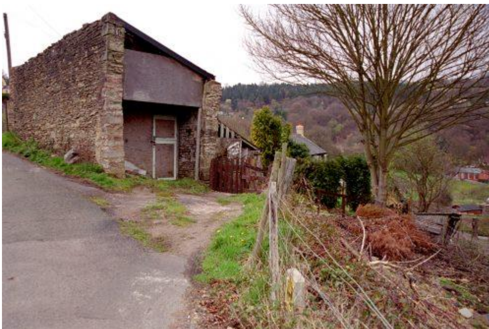
A distant view of the 'Deep level' site, looking E
