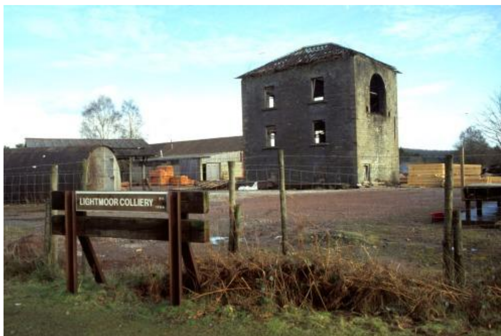
The former engine house (SO 642 121) looking SE
