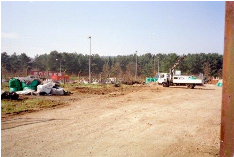
Bilson Colliery Site (3)
