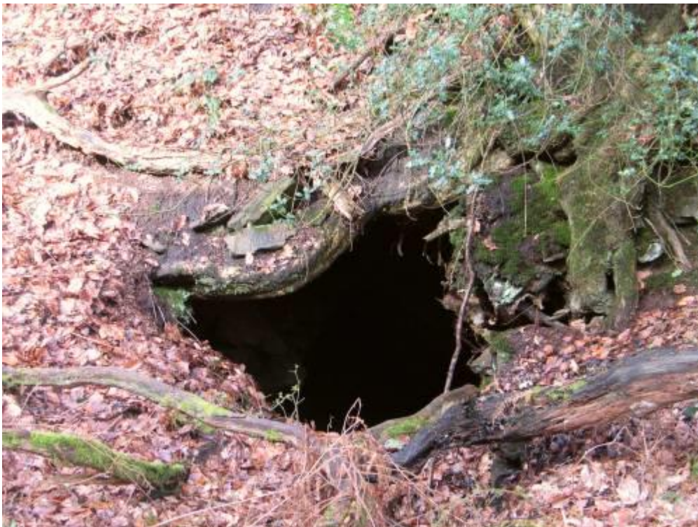
A second collapse (SO 6004 1151) looking NW
