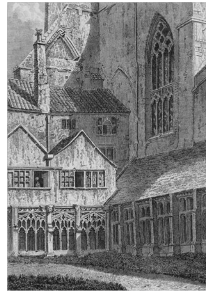
Now demolished Minster House & part of the cloisters at Bristol Cathedral
