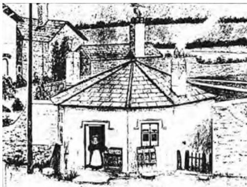
Sketch of the former toll house at Lydney (long since demolished), which was located opposite Bream Road adjacent to Tesco petrol station
